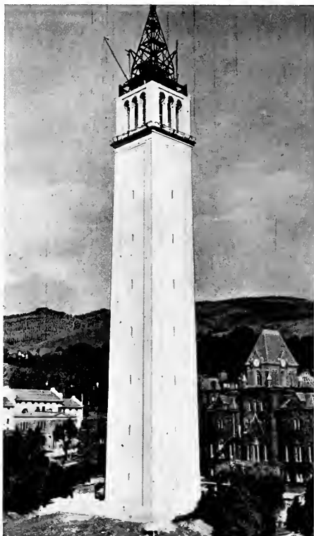
SATHER TOWER, UNIVERSITY OF CALIFORNIA, BERKELEY, CAL. JOHN G. HOWARD, Architect
